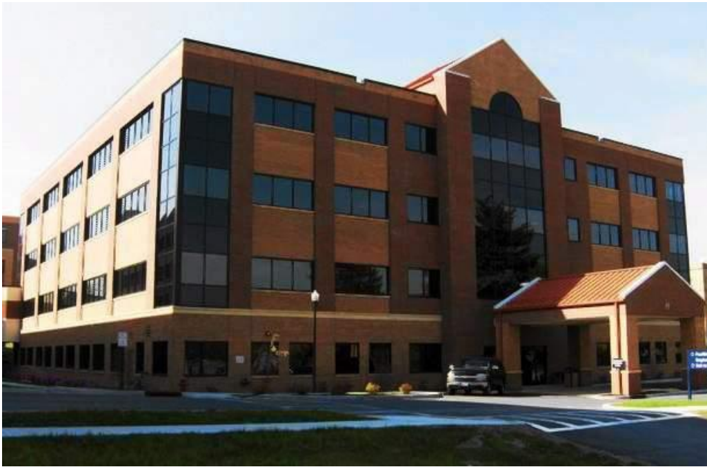
Part of St. Francis Hospital in Poughkeepsie Photo from www.sfhospital.org
